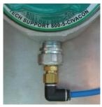
ASA-1 Pressure Switch mounted in ROM Overfill Socket
